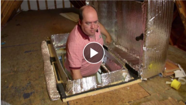
**Tri-County EMC: Energy Tip: Attic Insulation & Hatch Covers**
